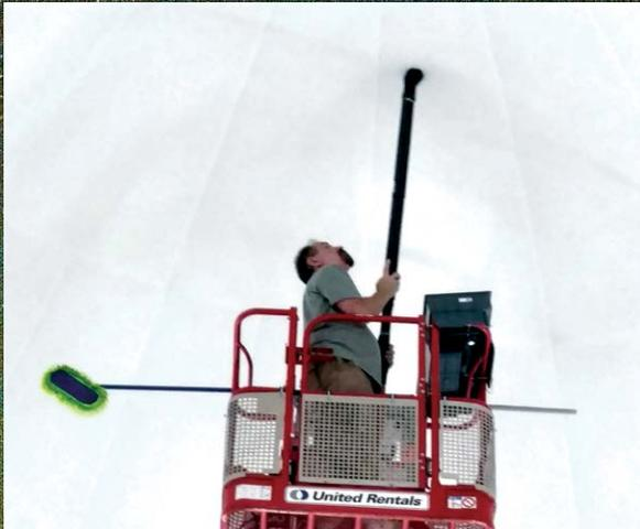
*Mark Perkins of Free Fall Technologies of Grand Rapids carefully vacuums the dome to remove dust that has accumulated on the dome and in the tiny perforations.*
