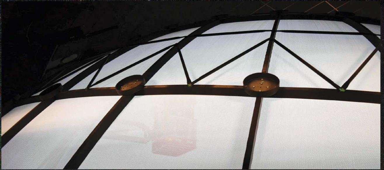
*Our planetarium dome is an assembly of 197 perforated panels that contain nearly 7500 tiny holes per square foot. Note that one of the lifts can be seen through those tiny holes from the back side of the dome.*
